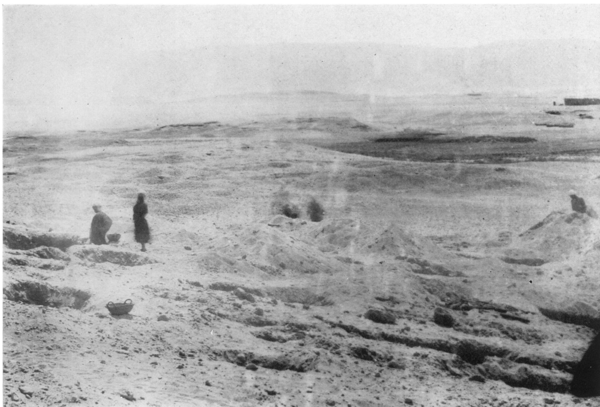
1. View of the work looking east
